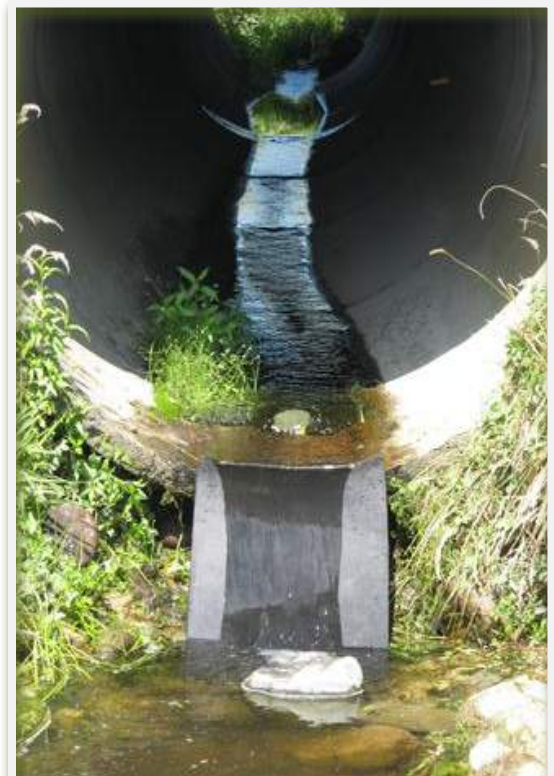
The photo shows a remediation job undertaken two years ago in the Aorere Catchment of Golden Bay. Large schools of inanga are now found upstream of this culvert whereas there were none previously. After two years this conveyor belt material is covered with bryophytes and looks natural.
