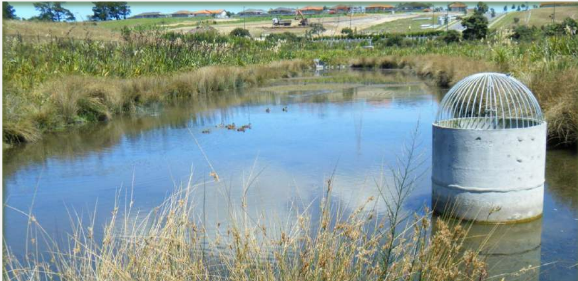
Stormwater pond near a new subdivision in a development hotspot, Westgate, Auckland.
