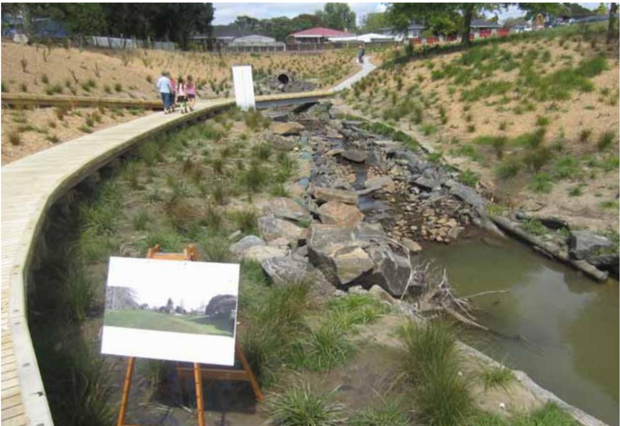
La Rosa reserve southern stream after culvert removal, daylighting and subsequent riparian planting and boardwalk construction
