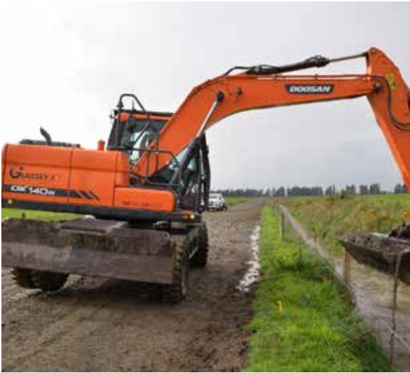
Digging sediment trap Living Water, Oct 2020. Photo © Jon Harding
