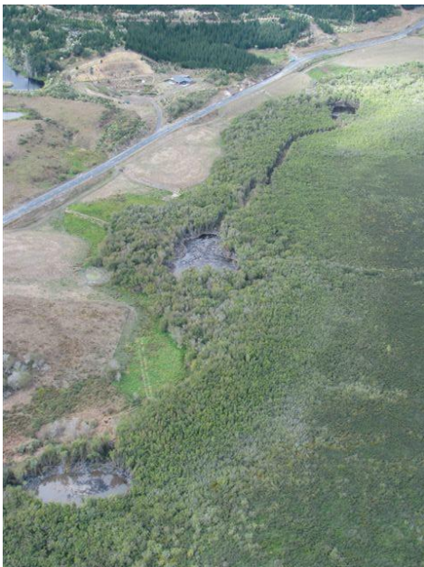
Coalfields Road project on the edge of the Whangamarino wetland
