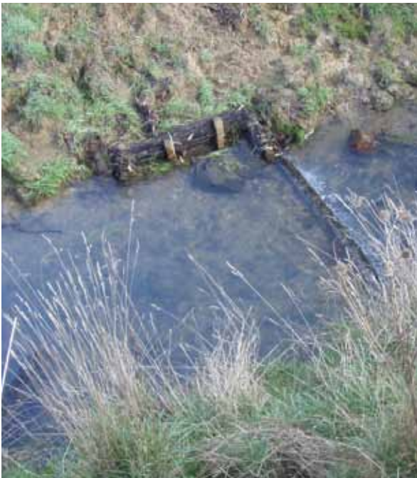
Sill log with bank armoring modification at the upper Keripaka Stream site, Whatawhata.
