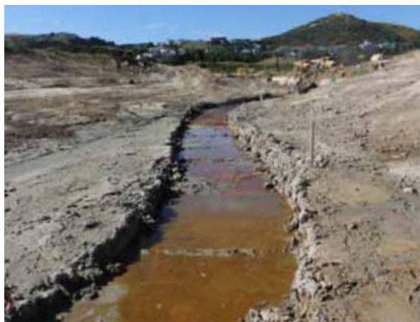
Duck Creek under construction.
