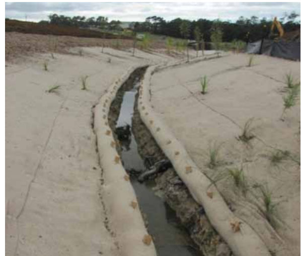
Constructed stream reach at Riverhead, showing recycled instream habitats of root bundles and logs.
