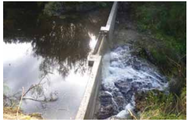
Trout barrier recently installed in Akatore Creek (cost 20k, including consents).
