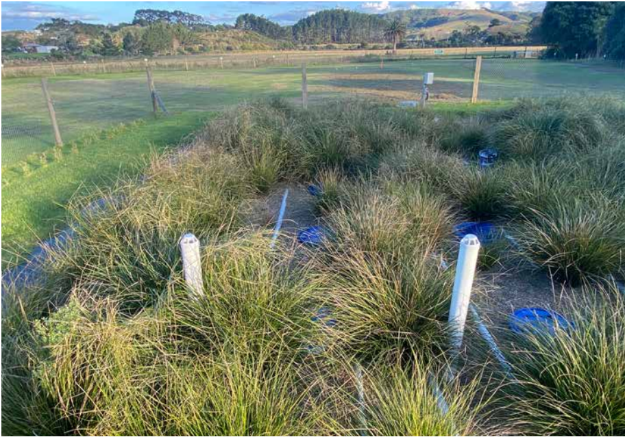
Project: Focus on ecocultural wastewater treatment systems. Multi-layered vertical flow constructed wetland treating wastewaters at the Te Kopua Whanau Campground. Photo: Chris Tanner/NIWA.
